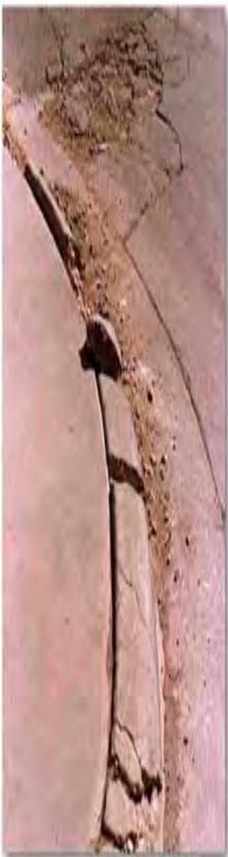
This un conventionally-shaped curb and the adjacent street have sustained substantial damage and deterioration.
