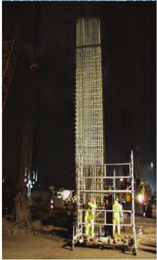
GFRP rebar cage being prepared for installation of the soft-eye.
