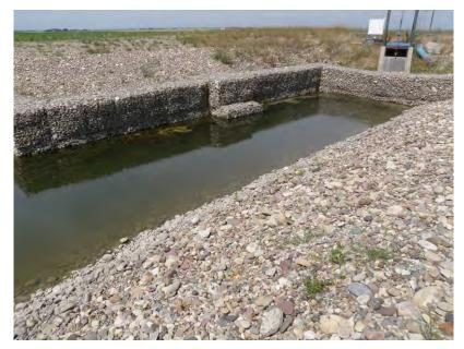
The Chin Lateral 7 Settling Pond was observed July 22, August 6 and August 11 during the irrigation season. The highest loading is shown in these photographs and was observed on August 11<sup>th</sup>. Both aquatic weed and filamentous algae mats are present on the upstream side. The Water Coordinator indicated that the total growth of aquatic weeds and algae was similar to
