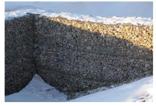
There was only one area of the Chin Lateral 7 structure that had excessive bulging due to a longer than 1m long cell used on a custom fit to the bank.
