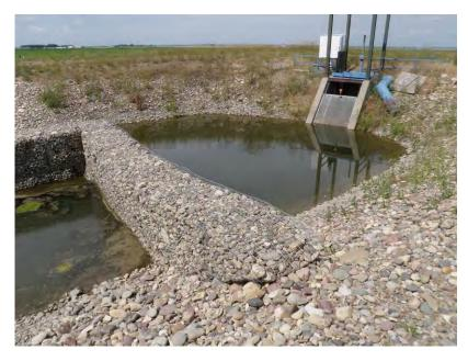
In this second photo the distinct change in presence of aquatic weeds and algae on either side of the wall is observed. The fine screen on the inlet structure was in place during the entire irrigation season with no accumulation. Irrigators reported to the Water Coordinator that the gabion wall "is a blessing to them" and that they are not needing to clean their on-farm pressure filters very often compared to previous years.
