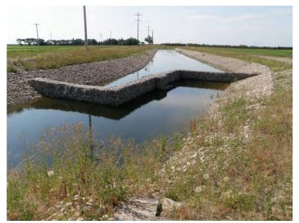
There were two days of during the 2010 irrigation season during which the Chin Lateral 7 system was operating near design flows. The Water Coordinator indicated that during this time aquatic weeds and algae that were growing in the canal was being transported to the gabion wall. There was no measurable difference in the water level on either side of the wall, indicating negligible hydraulic restriction with low weed loading.
