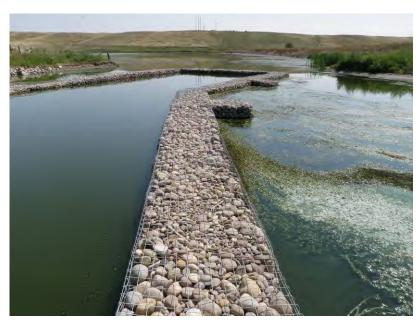
Due to high runoff, both pumps were operated through the entire 2010 irrigation season. At maximum weed loading, there was no measurable difference in water level on either side of the wall. A careful inspection along the wall revealed that inflow was relatively uniform, indicating that flow was maintained through the weed mat. A high factor of safety was used in setting the design
