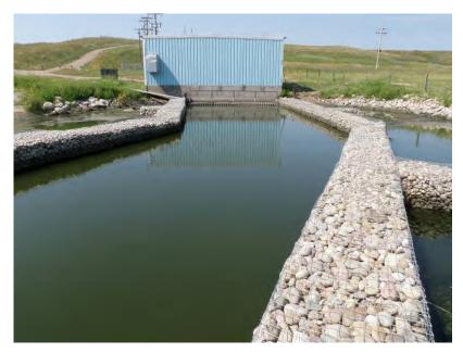
The Yellow Lake Pump Structure Inlet was observed June 29, July 22, August 5 and August 18. Screened sampling and qualitative analysis of the upstream and downstream water were completed once significant aquatic weed and algae loading entered the inlet bay. This photo shows the general configuration of the gabion wall infiltration system relative to the inlet.
