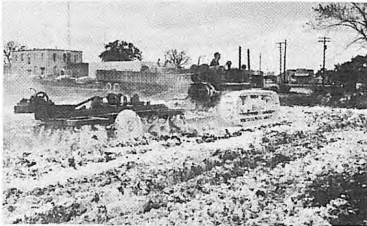
Lime is mixed into soil with twin disc harrow pulled by crawler tractor. Mixing starts right after lunch. 2:00 P.M.
