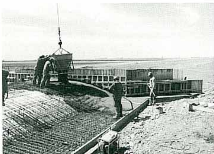
The seventy cubic meter concrete pour is completed in one day.
