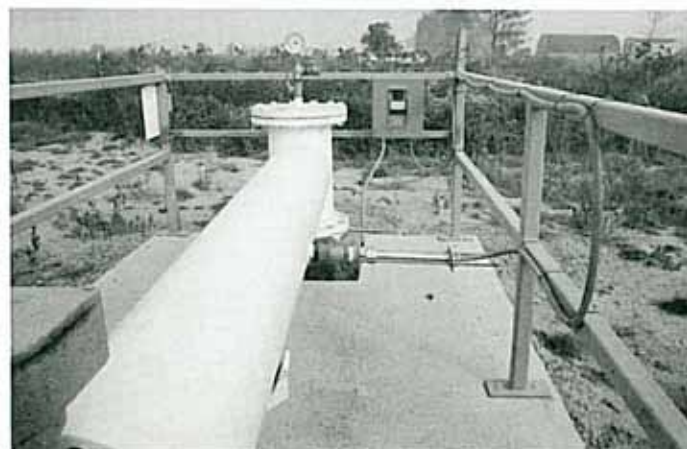
SMRID's Crystal Lake Lateral Pipeline. Each mag meter is calibrated for the size of pipe and again field calibrated to match flow conditions.
