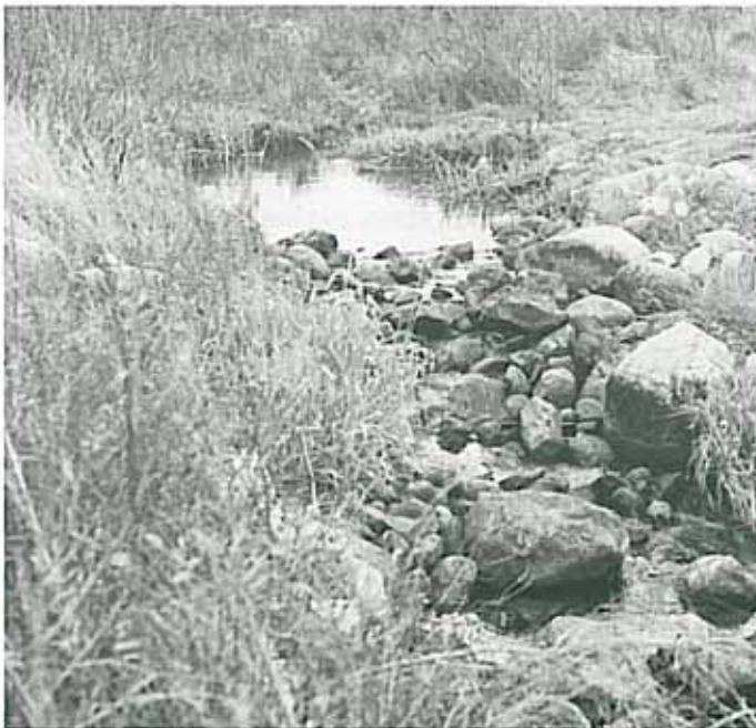
Rock drop in Drain 64 Hays has stopped erosion - excellent regrowth of vegetation occurring.
