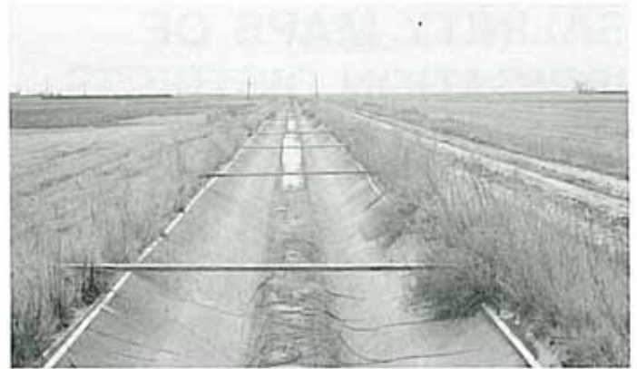
2 x 8's laid across lateral to allow side roll sprinkler to cross.
