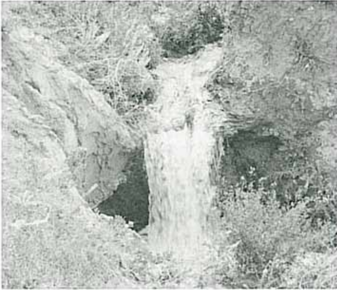
Erosion occurring prior to installation of the rock drops.
