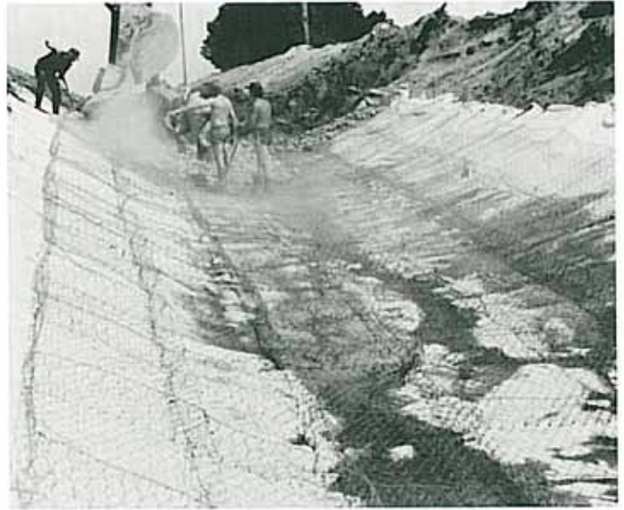
The wire units are filled by machine, however, some handwork is required to obtain an even placement of the rocks.
