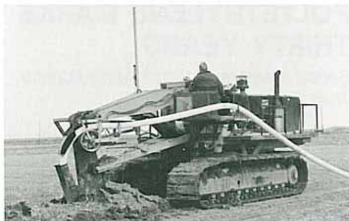
Wolfe plough is capable of installing drain tubing at a speed of 15 m/min.
