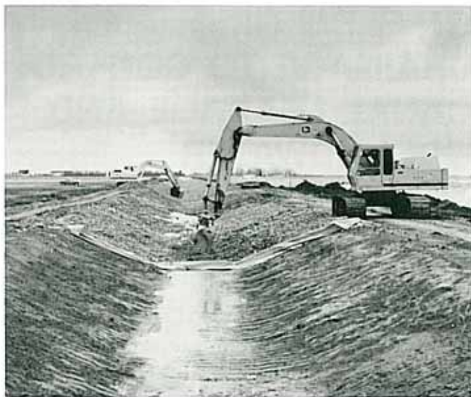
Screened granular backfill being placed directly on polyethylene lining (depth 300 mm).
