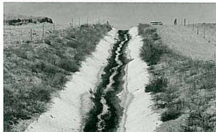
Below: Rehabilitated spillway (fabriform chute).
