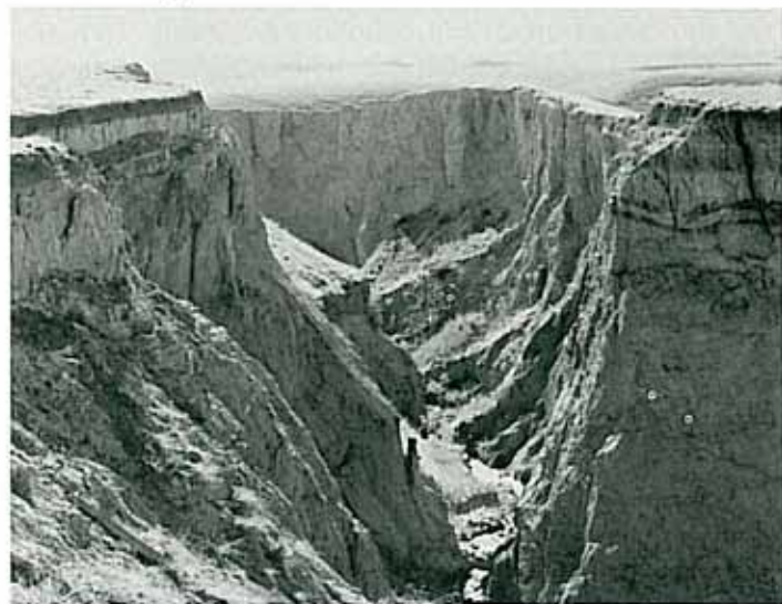
Above: Spillway in eroded coulee before rehabilitation.
