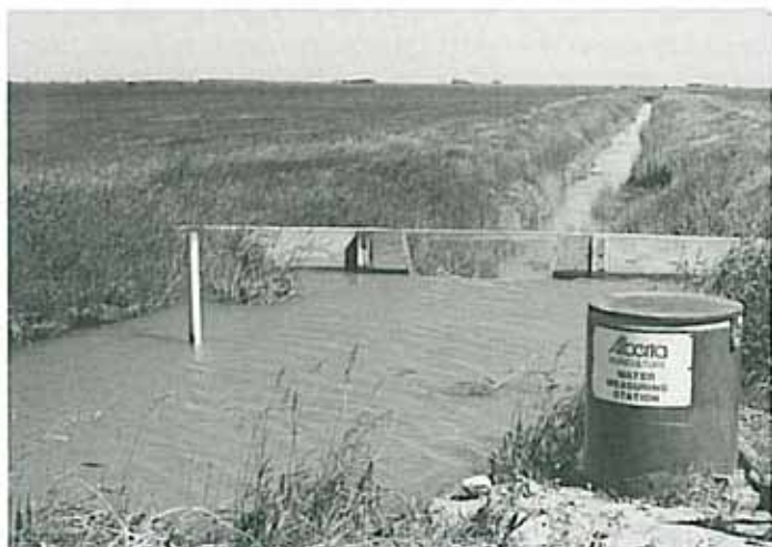
One of thirty-four typical Alberta Agriculture water measuring stations. This one utilizes a cipolletti weir.
