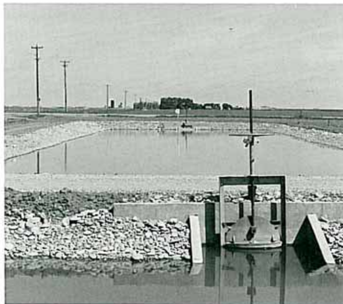
The settling pond constructed in 1989 on the S.M.R.I.D.'s Coaldale Lateral is lined and gravel armoured.
