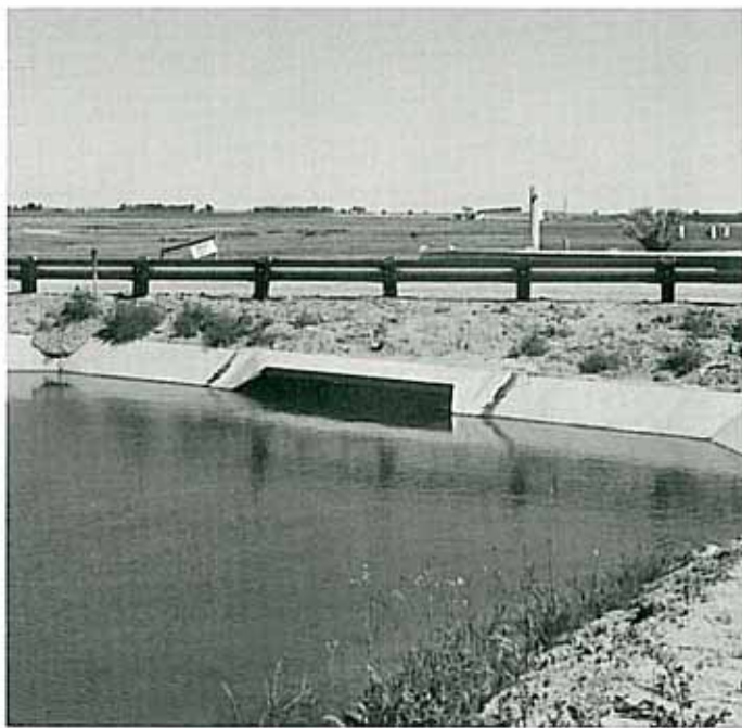
Note: Tranquil flow through the newly constructed box culvert (10 M 3 /s).
