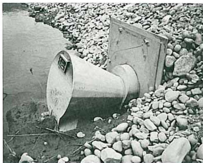
The Reg-U-Flow valve pictured above is installed on a 500 mm diameter turnout.
