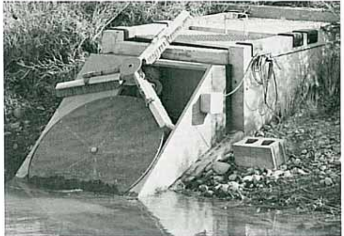
The electric driven rotating screen is actually a perforated disk, 0.9 m in diameter with three rotating brushes mounted on the top.
