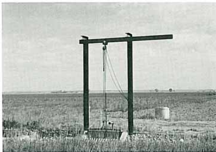
Gantry type hoists such as this one on the BRID's C6E Pipeline are considerably more costly.
