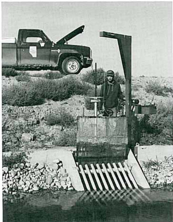
Assistant Water Master, Emil Johnson, demonstrates ease of removing and cleaning screens with new low-cost hoist.
