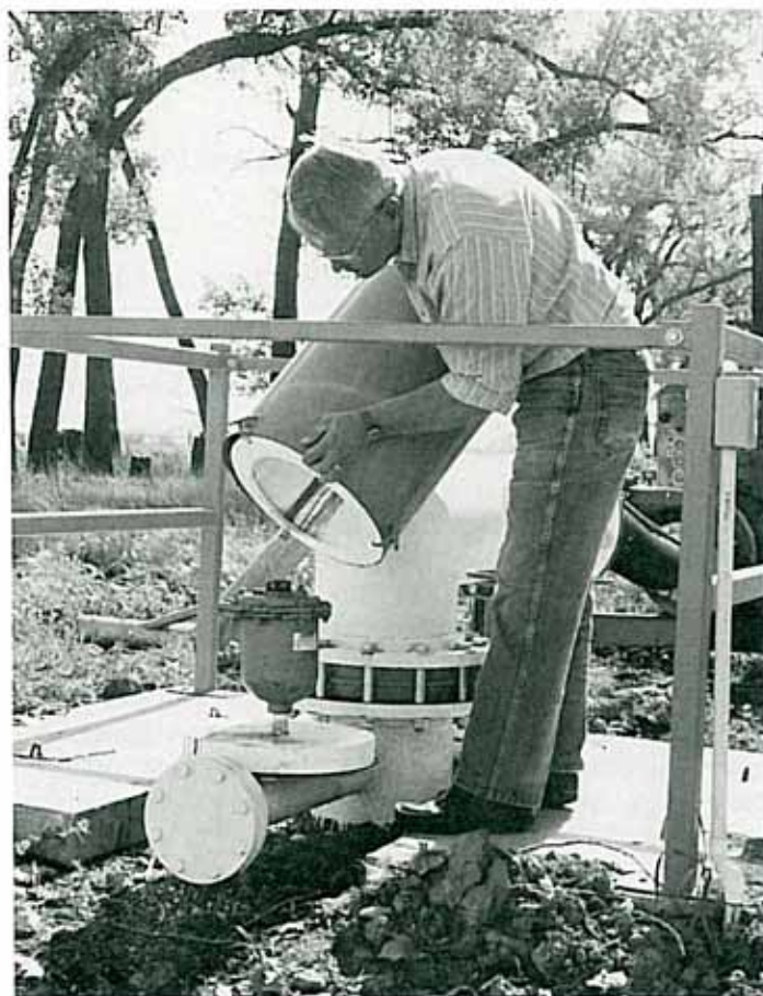
Technologist, Paul Ewashen, demonstrates how easily an insulated canister can be removed for valve inspection.
