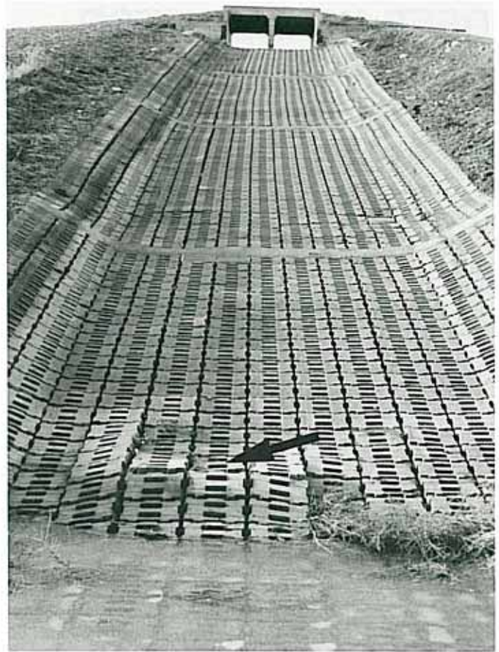
Note: Arrow points to blocks that have lifted due to the action of the hydraulic jump.
