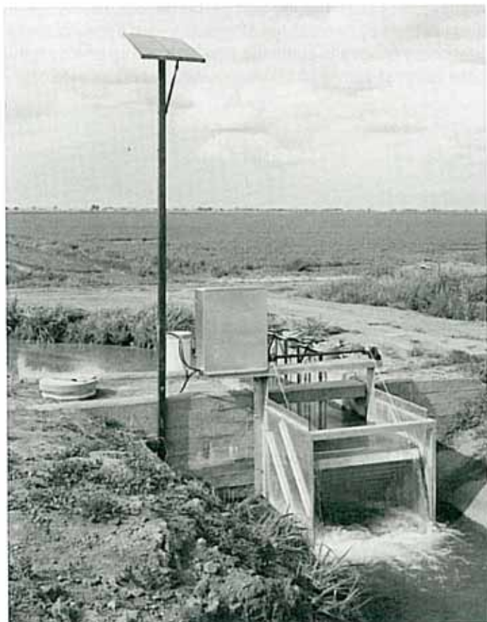
This smaller automated Overshot Gate is solar-powered but these gates can also be connected to the local electrical grid system.
