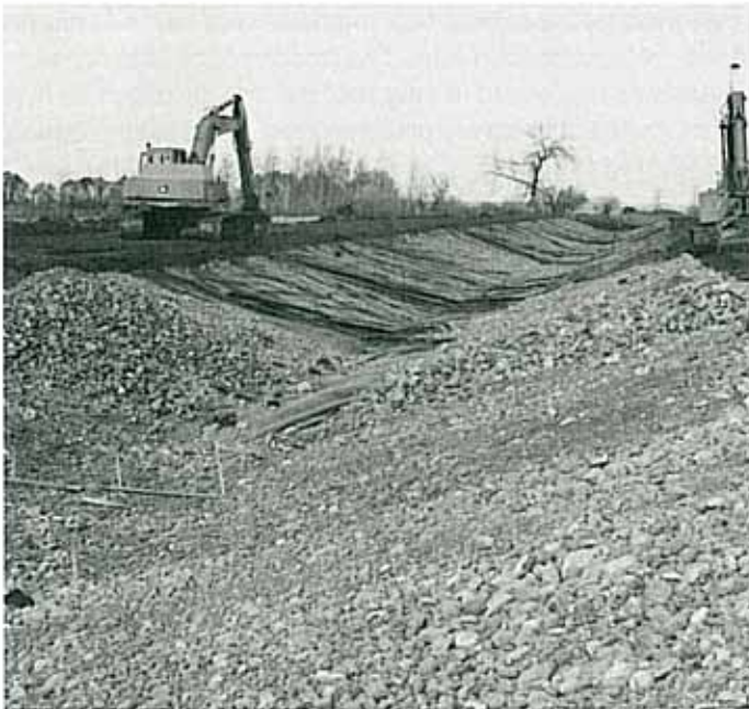
Woven polyethylene lining being covered directly by gravel armor.
