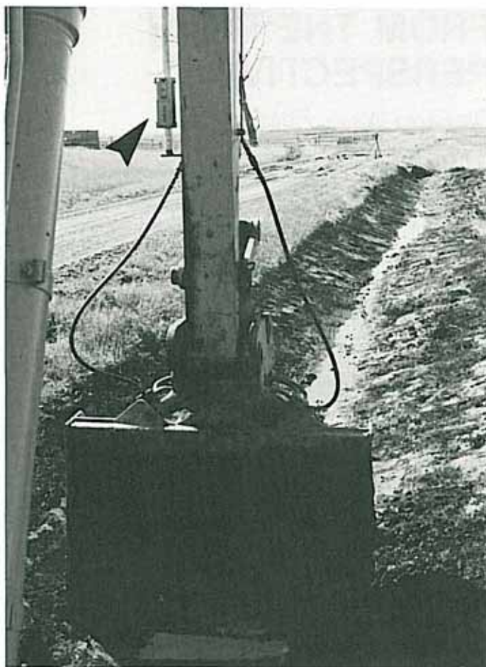
Arrow points to receiving box that lets operator know at a glance whether he is "on or off grade". Note: Laser Transmitter in background.
