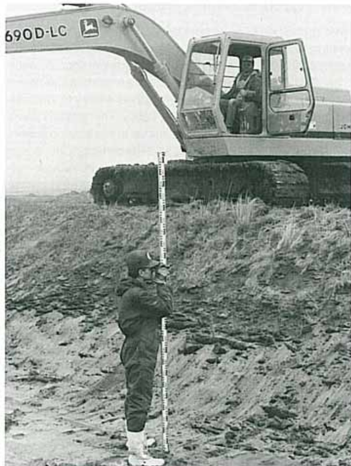
The "out-dated" rod and hand-level method.
