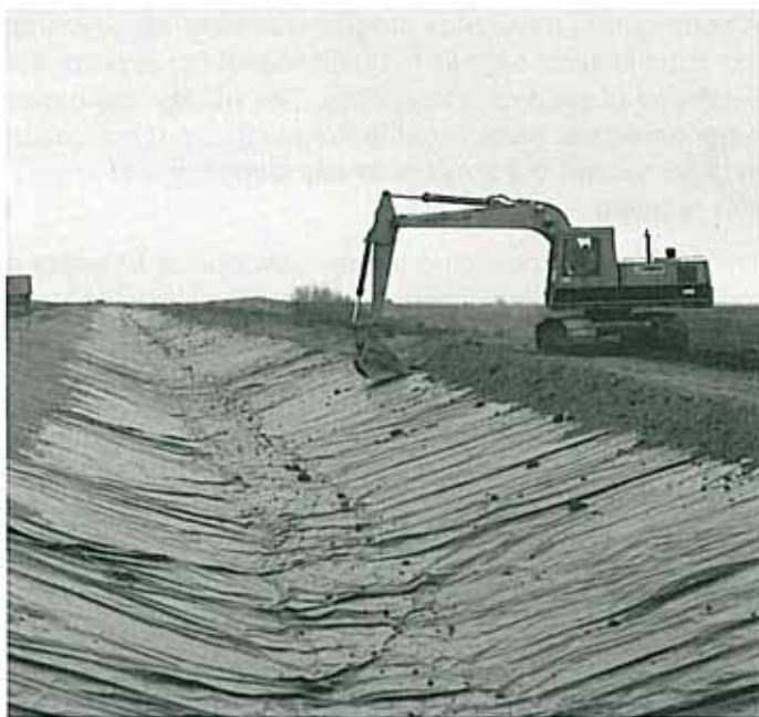
PVC canal liner being prepared for gravel armor.
