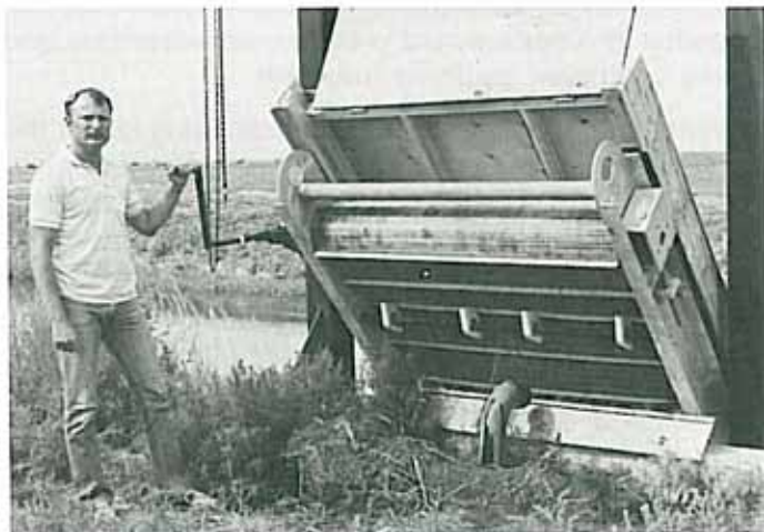
Steve Topping demonstrates the BRID's new rotating weed screen.
