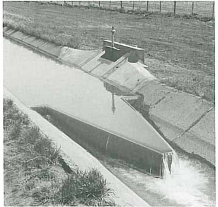
Duckbill weir installed on SMRID Six-Mile Lateral.
