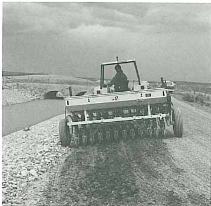
Traux Grass Drill seeding canal slopes (June 1990).
