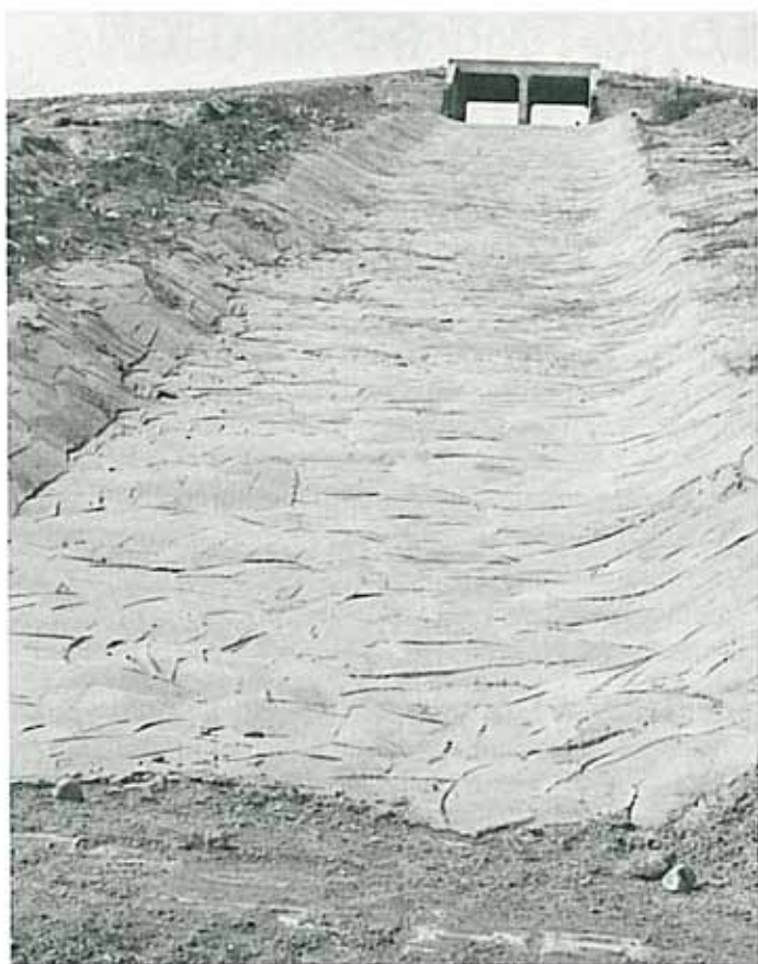
Spillway after sealing the surface and pumping grout underneath.
