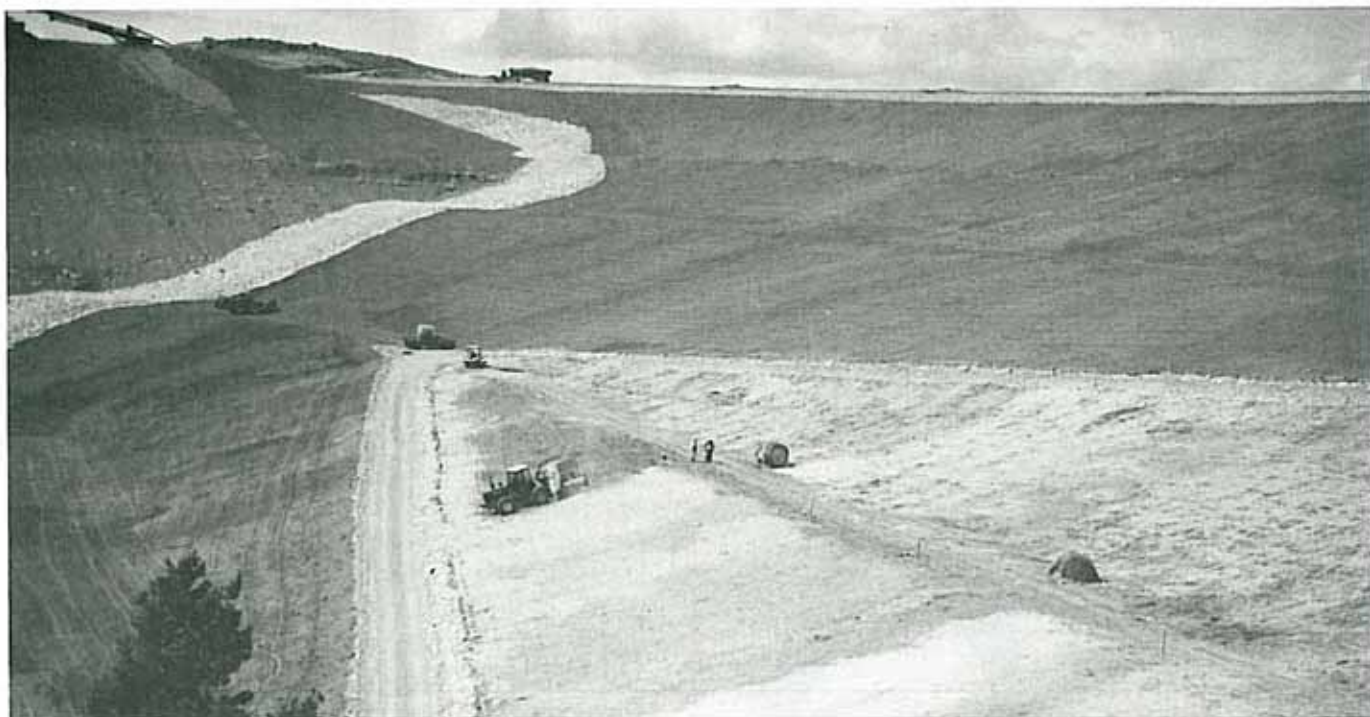
Overview of downstream slopes of Oldman River Dam. Light areas have straw spread and await Crimping.
