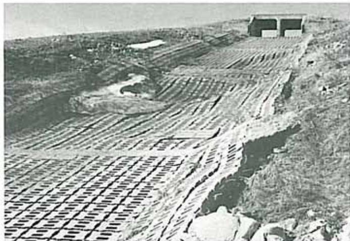
Note extensive damage to Bullshead Creek spillway.
