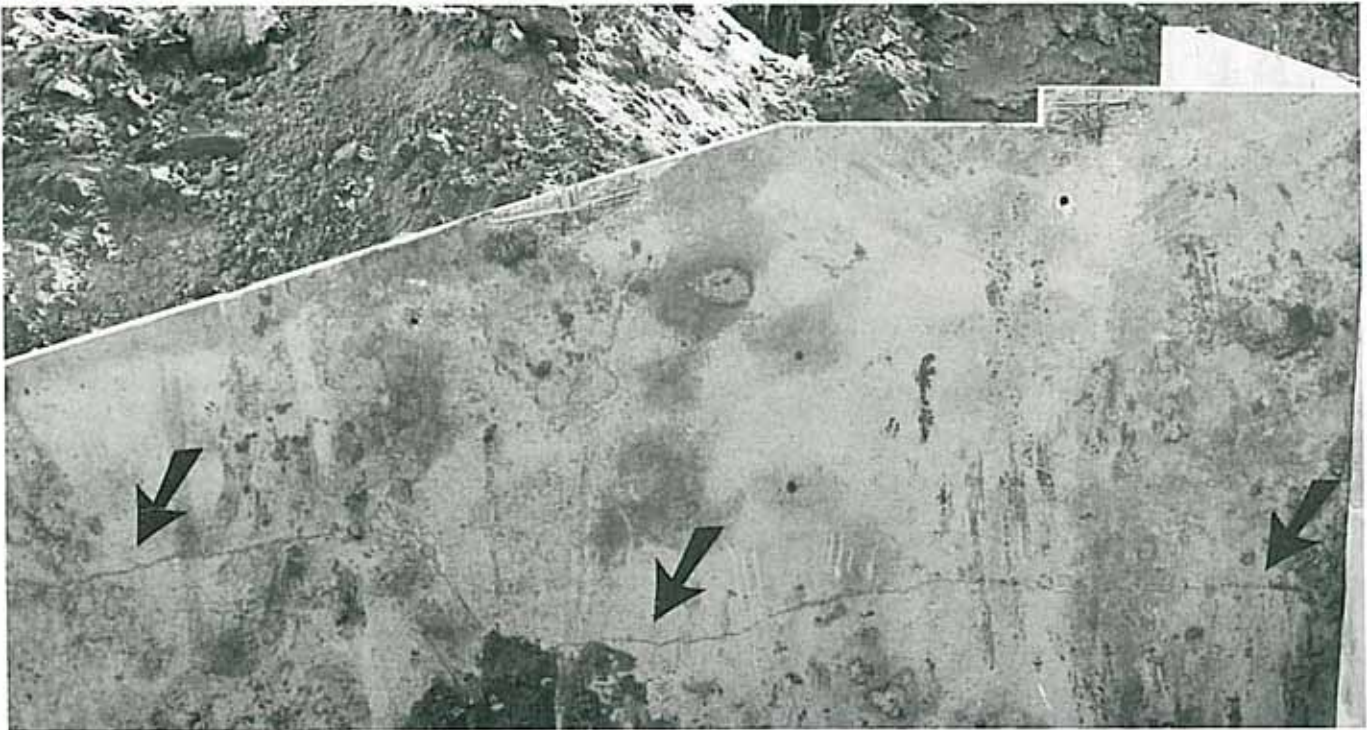
Arrows point to horizontal crack in large 5500 kg panel. Note: Missing lifting hooks that broke away during placement.
