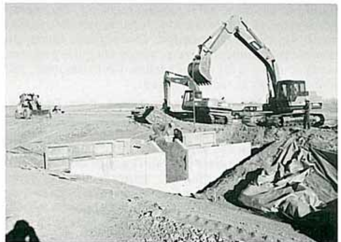
Large Precast Check-Drop Structure being assembled in polyethylene lined lateral.
