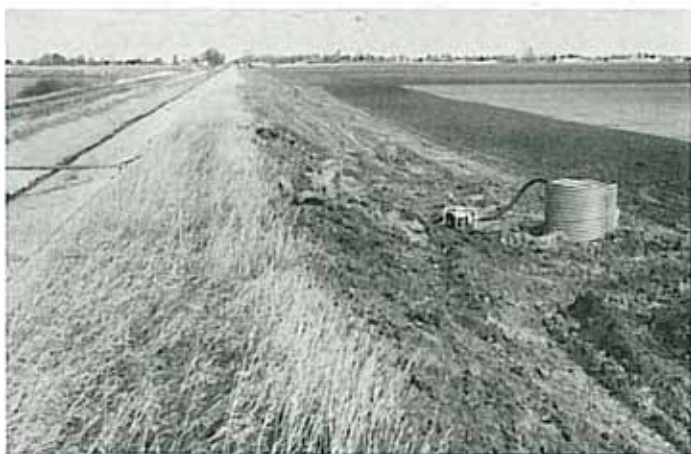
Portable pump at manhole (picture taken before submersible pump was installed).
