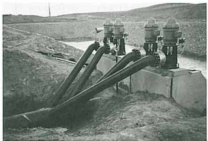
TID Lateral M's 40 Hp vertical turbine pumps.
