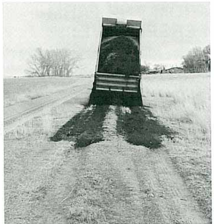
Spreading gravel to fill in wheel ruts on old driving bank.
