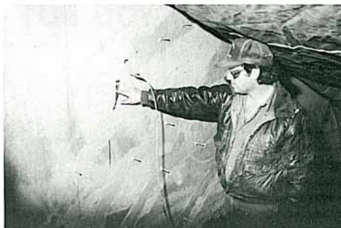
Dave Nolan of the BRID points to resin beginning to bleed from crack.
