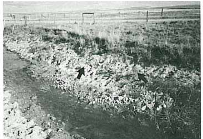
Arrows point to buried polyethylene lining that has been exposed due to cattle trampling earth bank when coming to drink.
