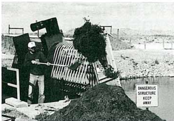
Emil Johnson forks weeds from holding pit. An automated conveyor belt will make this manual task unnecessary in the future.
