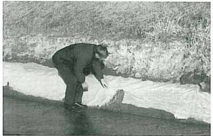
Allan Herbig, P.Eng., inspects damaged exposed canal liner.
