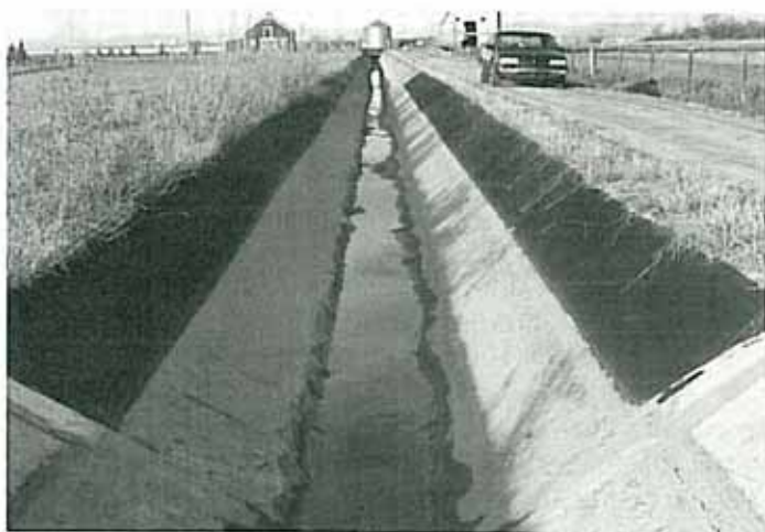
NOTE: Darkened area where Teranap 431 TP was bonded to concrete.
