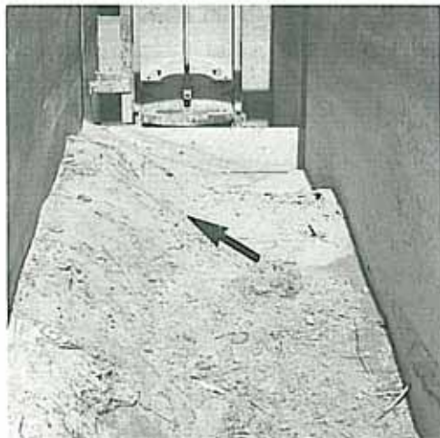
Arrow points to huge buildup of silt in front of stop-logs in SMRID main canal turnout.
