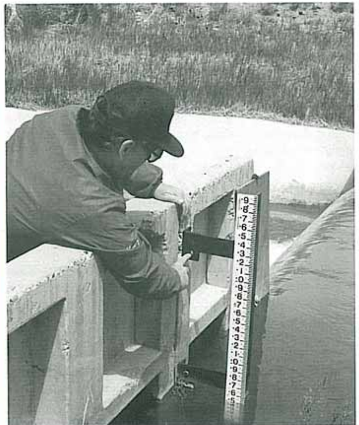
Larry Burr points to slot in bracket that allows vertical adjustment.
