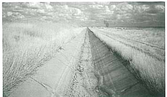
The 25-year-old SMRID Lateral #20B concrete lined lateral remains in good condition because of annual maintenance.
