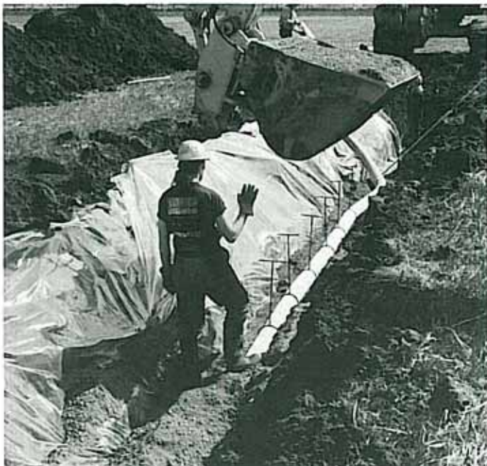
Alignment Forks placed 2 metres apart hold tubing in place while sand filter is placed.
