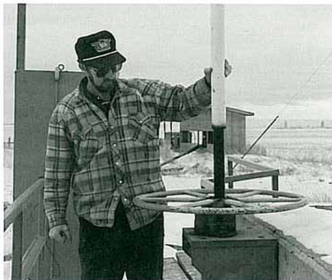
Ralph Oldenburger lifts gate stem cover from hand wheel gate.
