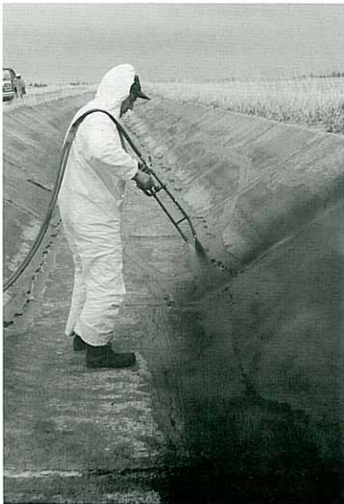
Liquid Boot being sprayed on test reach of the badly cracked Cameron Lateral.
