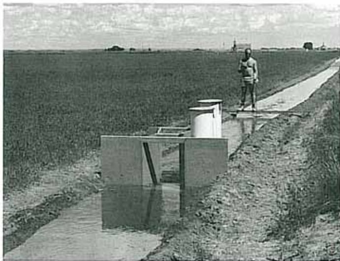
Technologist Lawrence Schinkel measures accuracy of Cutthroat Flume.
