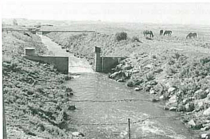
Flow metering station on open drain.
