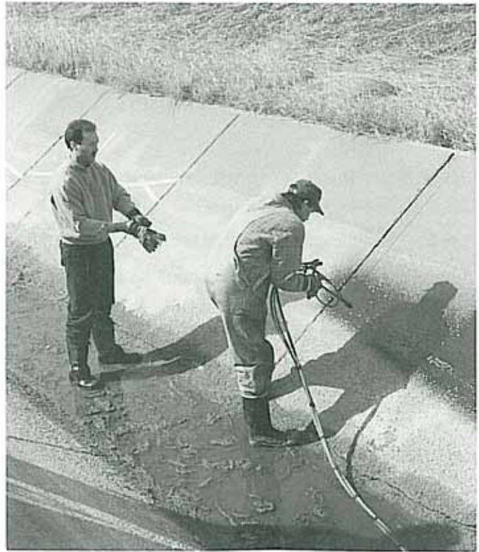
Armorthane® being applied over cracks in early spring at test site.
