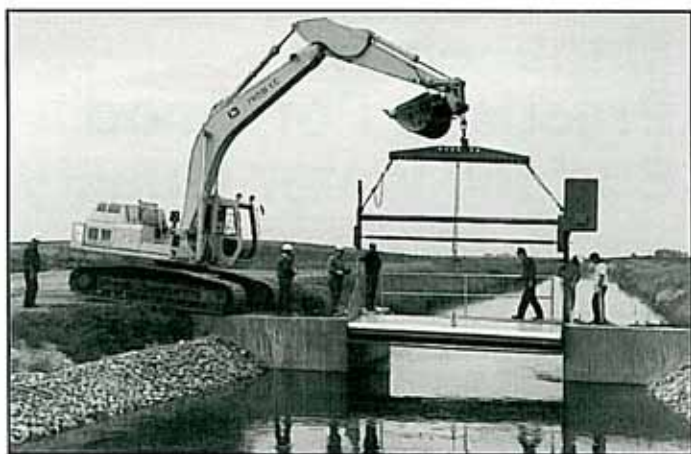
Hydraulic Hi-hoe lowers Langemann Gate into existing concrete structure on BRID's Lateral B. Note: canal is in operation.
