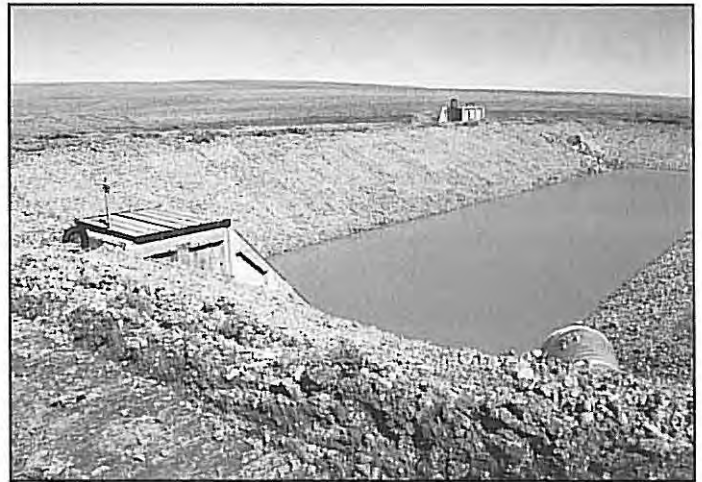
Lateral B1C settling pond is located parallel to canal.
