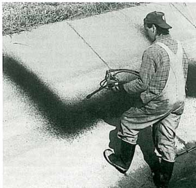
ArmorThane® being applied onto cracks on concrete-lined canal.
