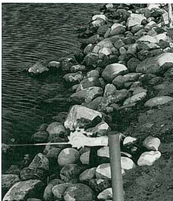
High tensile wire at 4-metre intervals across water.
