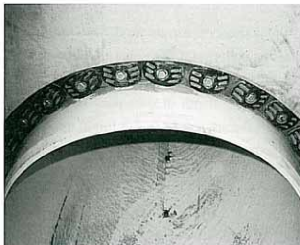
Seal assembly into space between pipe and wall.
