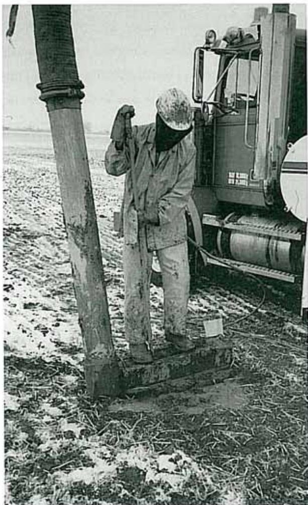
Hot pressurized water being sprayed through brush block as vacuum sucks out the slurry.
