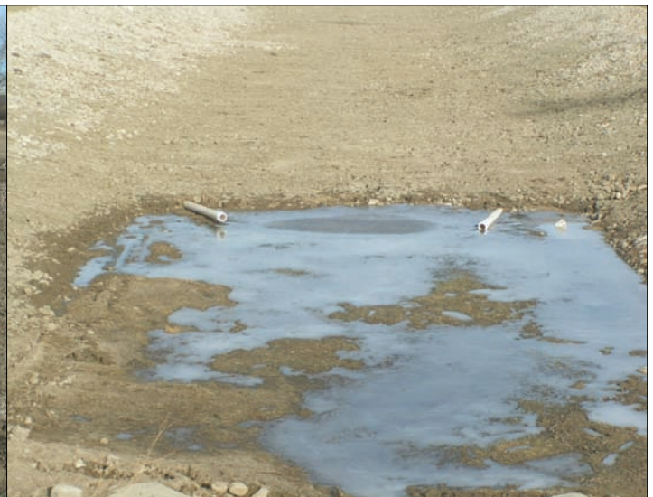
A section of PVC pipe was connected to the plastic drain tile at end of the liner to drain groundwater collected from under the liner.
