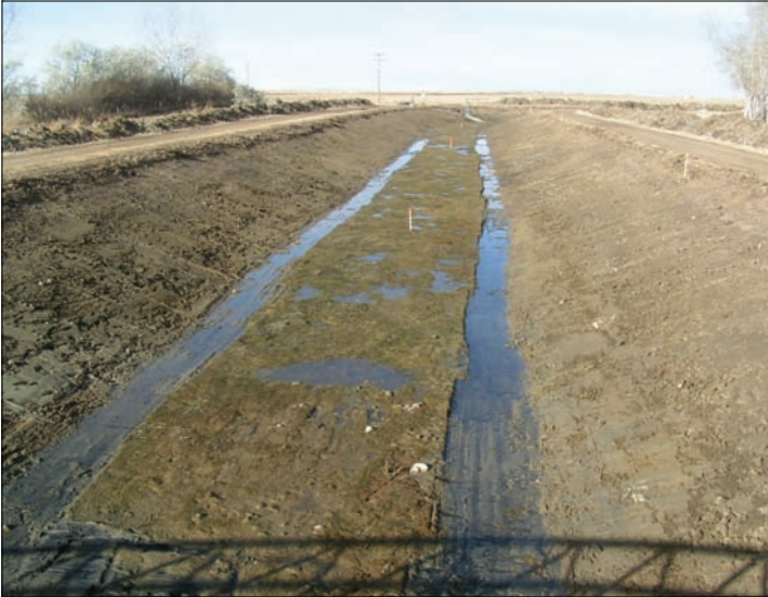
A shallow trench was excavated in each toe of the bed for placement of plastic drain tile.
