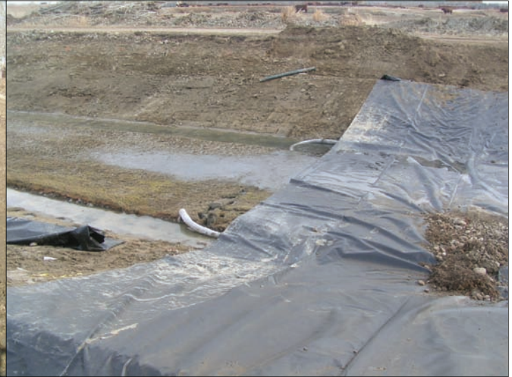
The plastic drain tile was placed in the shallow trench prior to installation of the canal liner.
