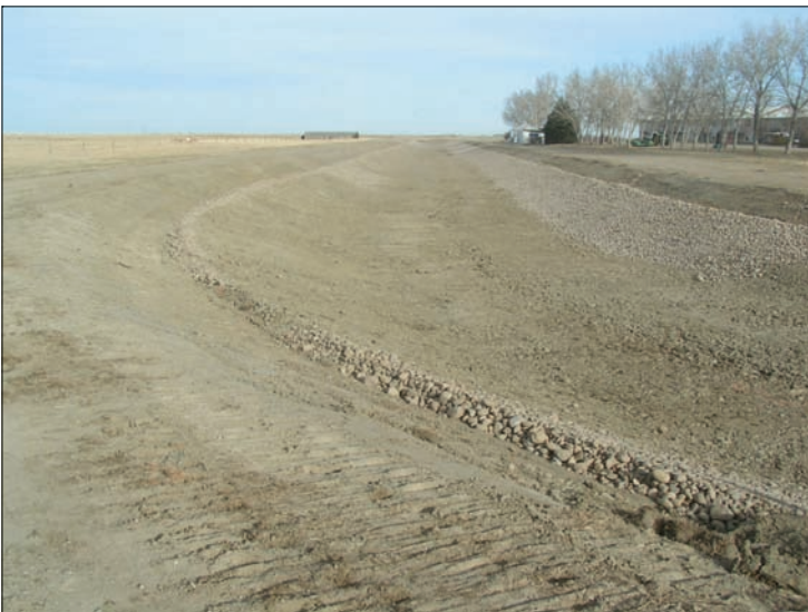
Armour placed on canal liner.
