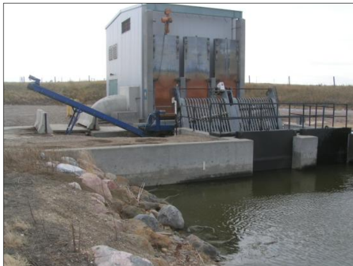
Pump house screens to be replaced
