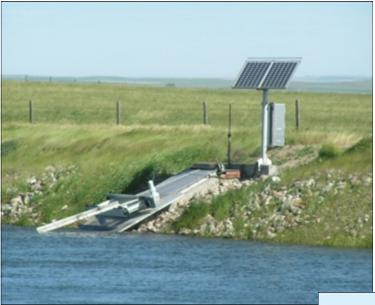
The screen is a 4.7 metre long x 1.6 metre wide stainless steel plate with  $\frac{1}{4}$ " round holes, with an open area of 40%. The smooth surface and small holes on the screen minimize the amount of debris caught on the screen, and make it relatively easy to clean.
