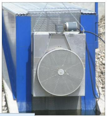
The WID designed the precast turnout structure with a basin deep enough to lower the screening unit into. An arm with a hand crank winch is provided to lower and raise the unit as needed for maintenance or just to keep it out of the water if not being used. The basin is situated below the canal bed meaning a check structure is not required in the canal to raise water levels and pumping units can be operated at low water levels.
